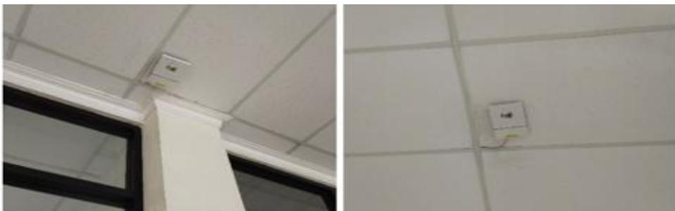
Gambar 100. AP Ruijie Terpasang di Wing Kiri dan Kanan Lantai 1 Laboratorium Terpadu
